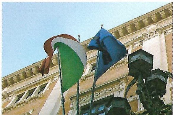
Views of exterior and façade of Palazzo Montecitorio.
